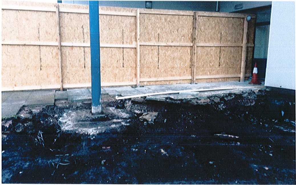
Exposed existing foundations to canopy
