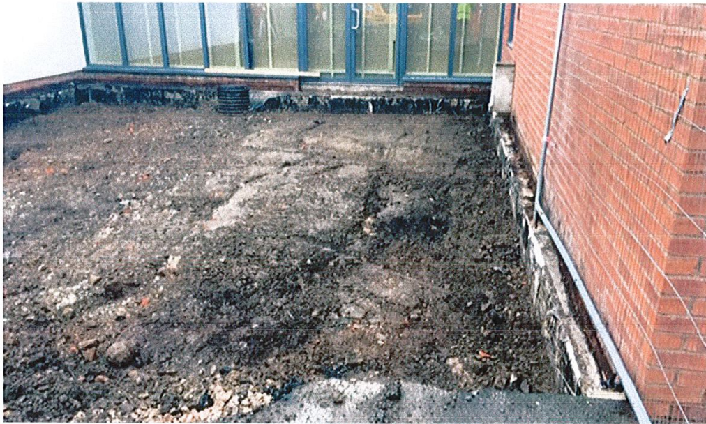
Courtyard area with slab removed
