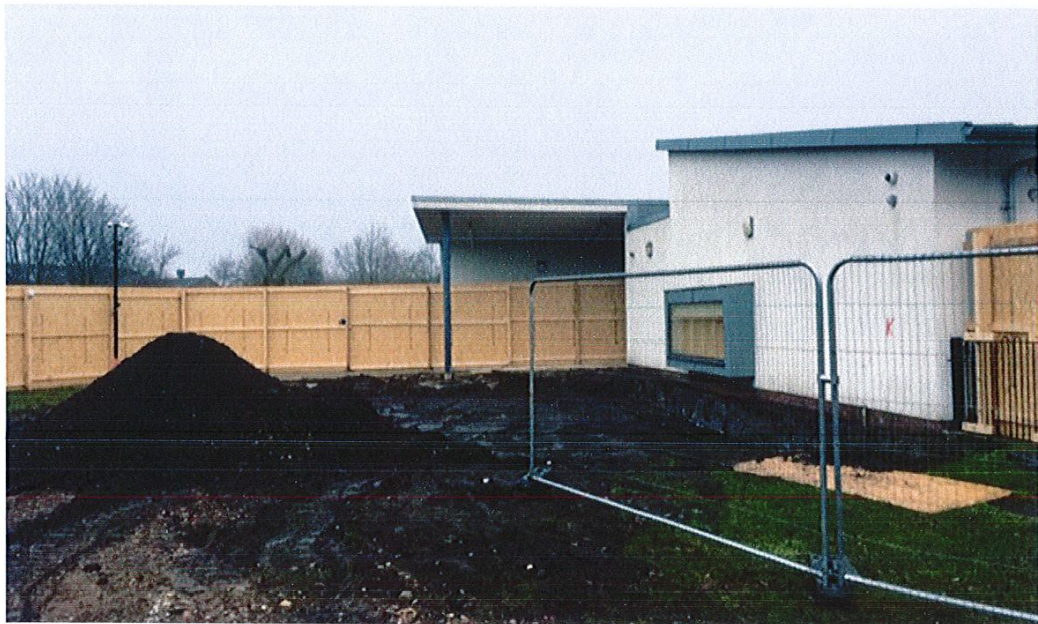
Further reduced level dig for excavations to new extension classroom including spoil heap from removal
